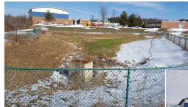
Before picture of a stormwater basin at Dallas Area High School
