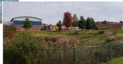
After picture of a stormwater basin at Dallas Area High School
