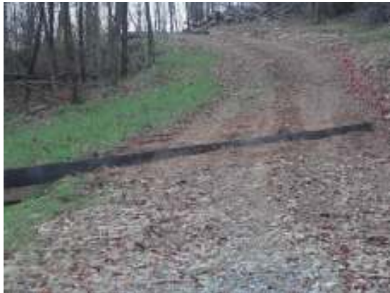
Completed Conveyor Belt Diversion
