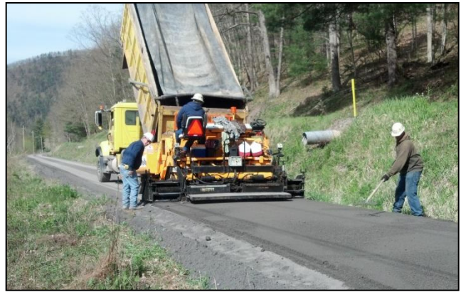
Paver-placement of TSA is preferred for longer sections of trail as pictured above.
